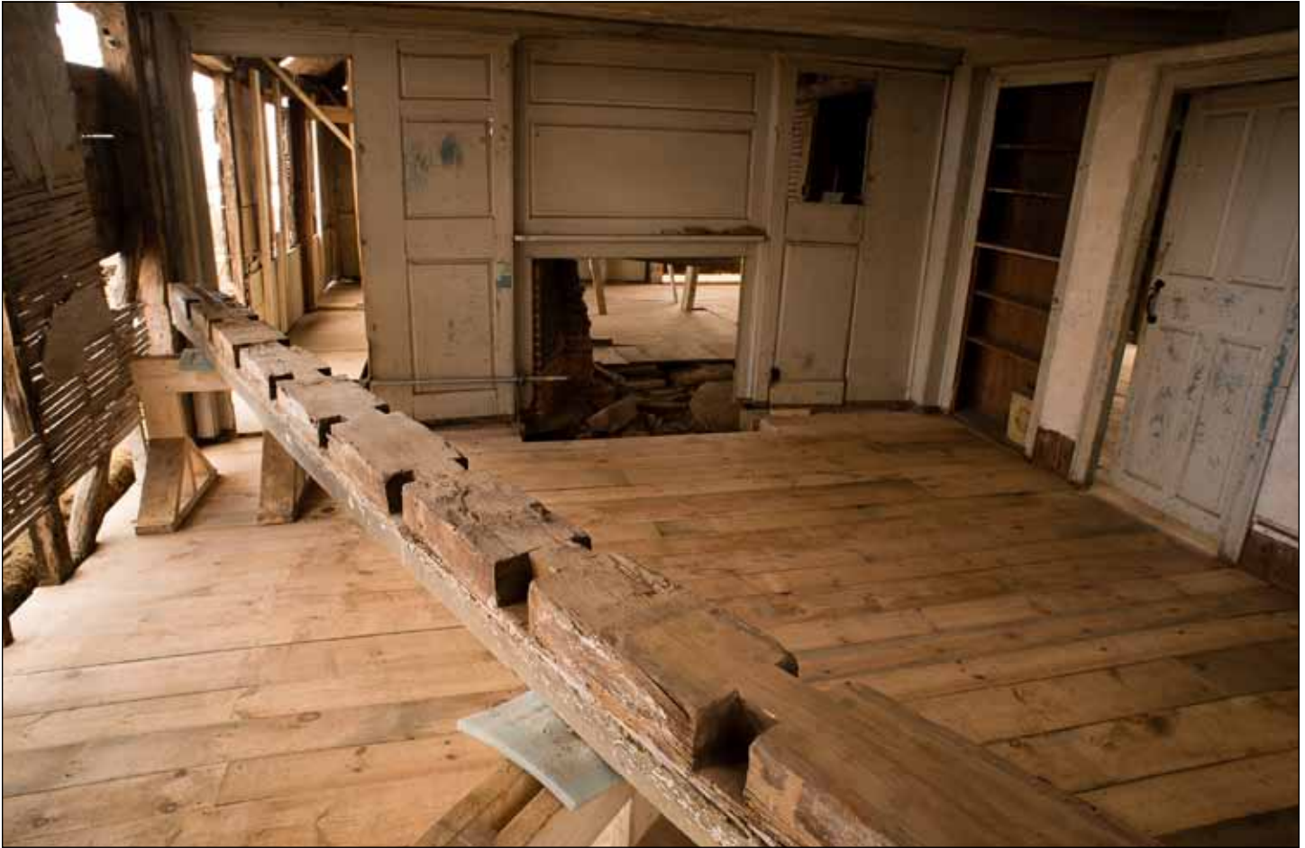
Original beam, carefully repaired.
