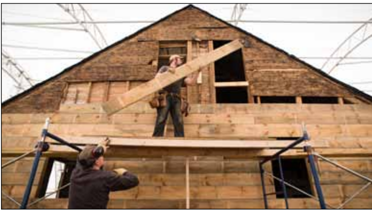
Sheathing the east gable.
