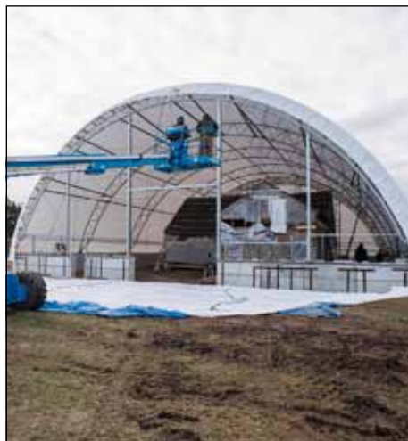
Restoring the Hancock-Mitchell House.
