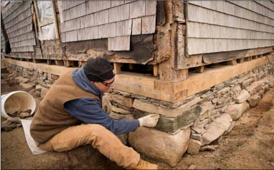
Creating the foundation.
