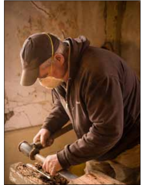
Mallet and chisel repair.
