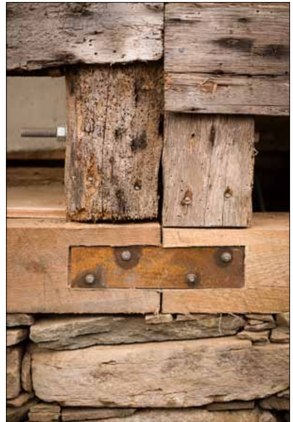
Old posts, new sills.
